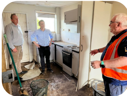
Site visits after the floods with
