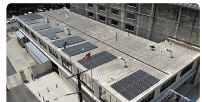
Rooftop shot of Solar Garden panels above Lismore office
