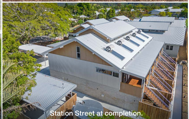
Station Street at completion.
