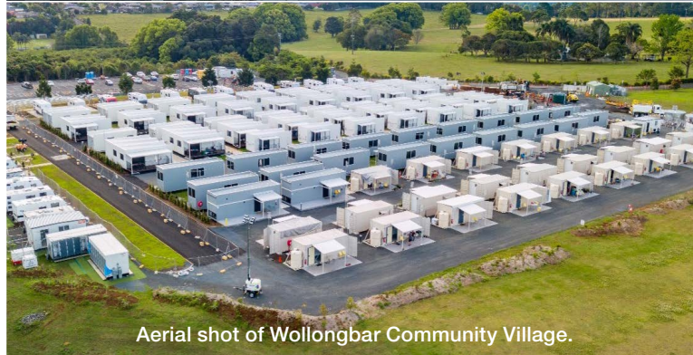
Community Village during construction.
