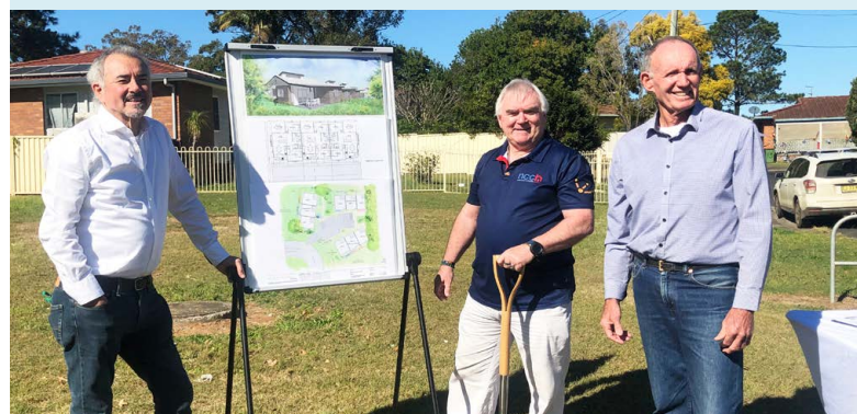
(L to R): Chris Gulaptis MP for Clarence with John McKenna & Rob Mustow at Callistemon Street, Casino groundbreaking.
